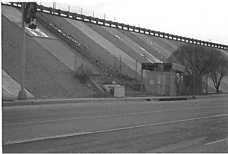
Illustration 4. Photograph of the pump station on Maloney Street. This pump is maintained by the New Mexico Highway Department as part of the flooding reduction program. Behind the pump station is a raised portion of Interstate 40. This construction acts like a dam and prevents drainage of water into the Puerco River, which is on the other side of the highway. During the flooding of 1998 the water reportedly got to a depth of 4 feet at this location.
